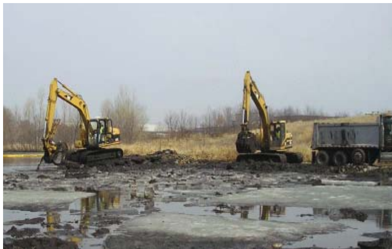
Photo 2: Excavators Performing Winter Dredging
