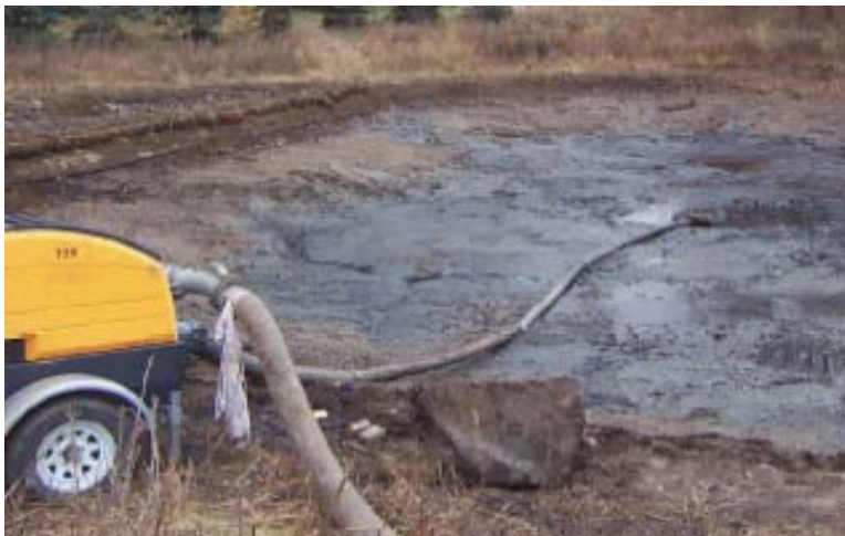
Photo 5: Pumping Equipment Dredging from Shore
