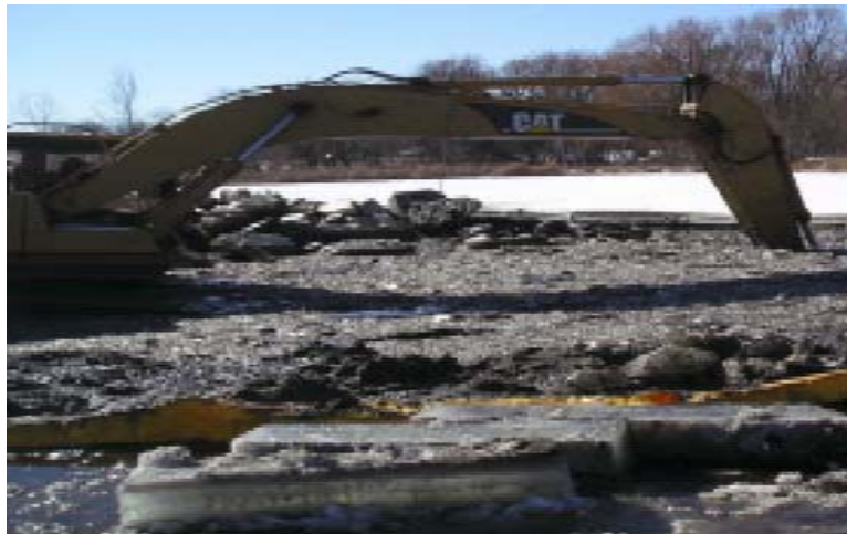
Photo 1: Excavator Performing Winter Dredging
