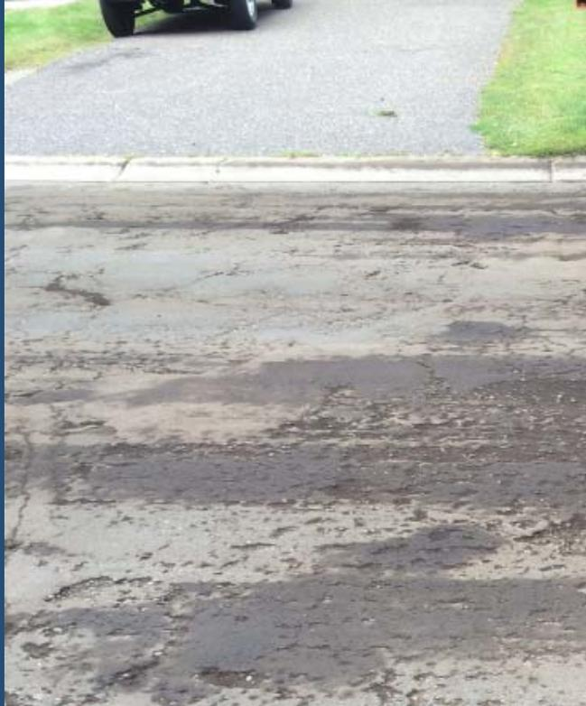
Photo of Pavement Stripping Failures
